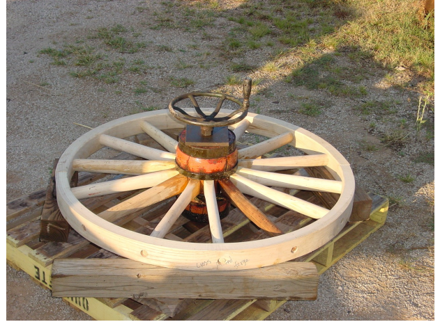
#7 Wheel blocked and secured for setting tire.
