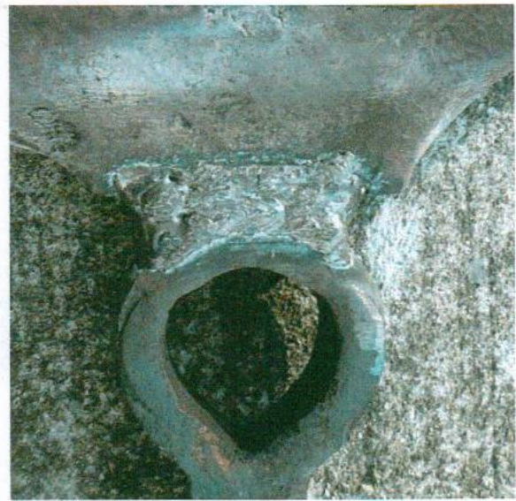
Figure 4: Anvil welded to post.
