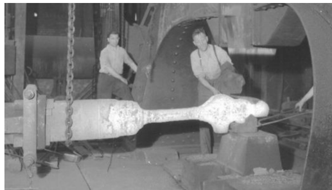
A photo taken in the mid 1950s shows workers positioning an ingot in 10-ton, double-column steam hammer to forge a locomotive connecting rod.
