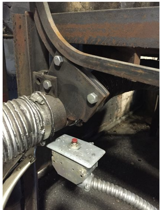
Air Gate Open and Fan Switch in "ON" position. Airflow is Adjusted by Gate Position.
