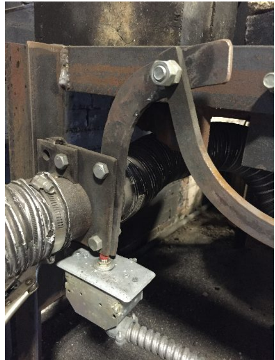
Air Gate Closed and Fan Switch in "OFF" position
