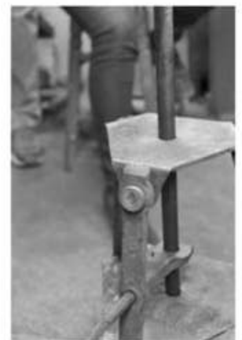
Setting the tenon in the square hole.
