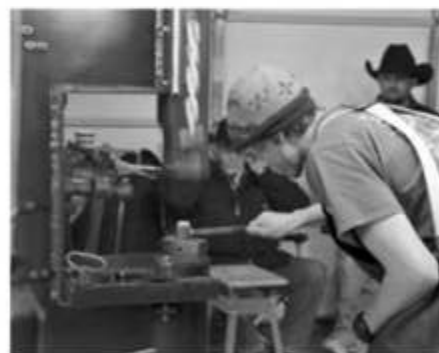
Heading rivets.
