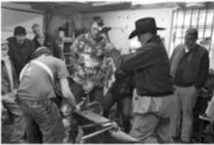
Setting the rivets.
