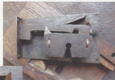
Right: Stock lock works; detail of interior.
