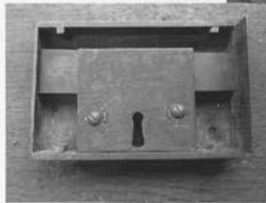
Right: Stock lock works; detail of interior.
