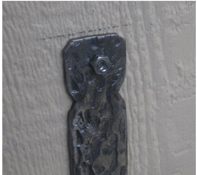
Photo 3: Distressed Lag Bolt
