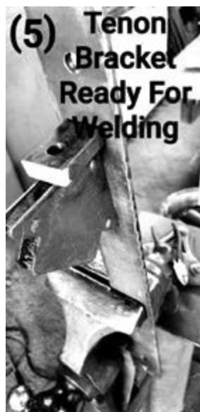
Tenon bracket ready for welding
