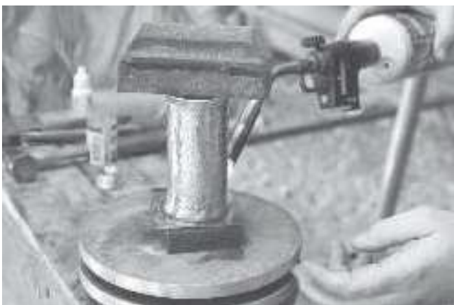
Heating the cup to melt the solder and get it to flow into and along the joint
