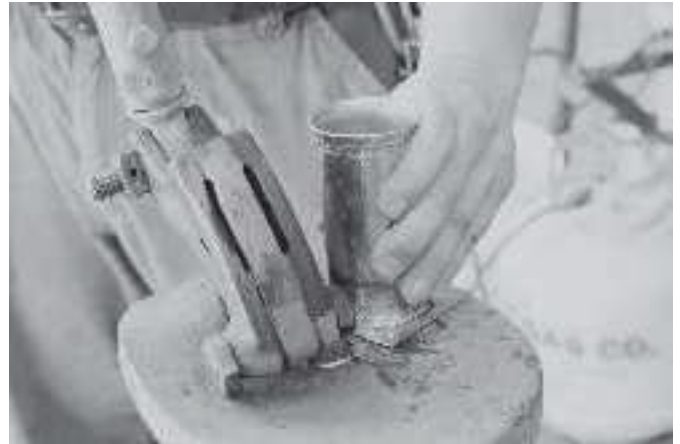
Trimming the bottom nearly flush with the bottom of the pipe
