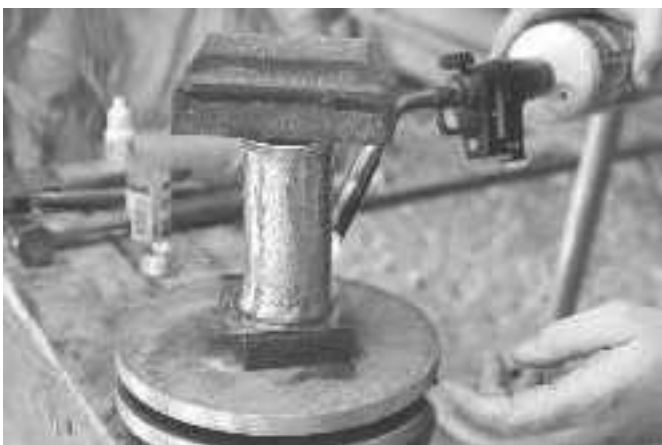
Heating the cup to melt the solder and get it to flow into and along the joint
