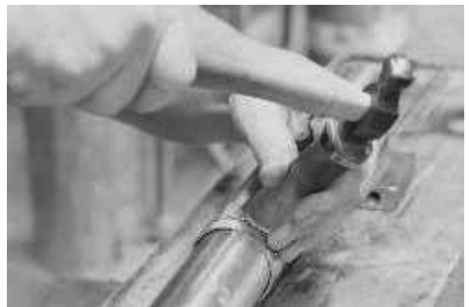
Below: Going over the chasing with a wider tool
