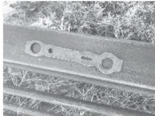
Above: Round-punched and drifted hole on the left, slot-punched and drifted hole on the right.
